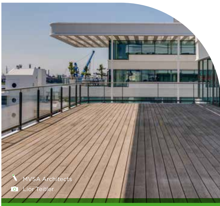
Jumbo Head office photo taken 5 years after installation (27,000 sqft) Schiedam, The Netherlands
